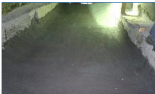
Completed application on a channel
