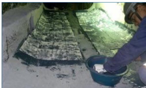
Belzona 9811 being applied on a channel
