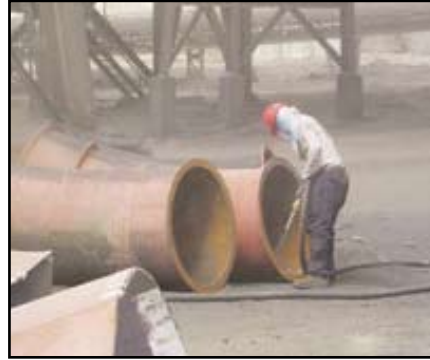
Agressive blasting surface preparation in process
