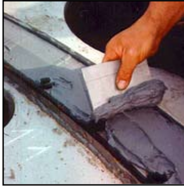
Application of Belzona® 1111
