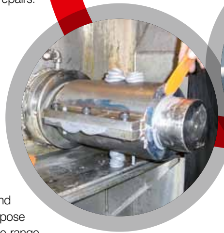
In-situ Shaft Forming
