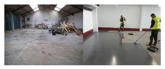
[Image 3- Disused warehouse before application] [Image 4- During application of the Belzona system]
