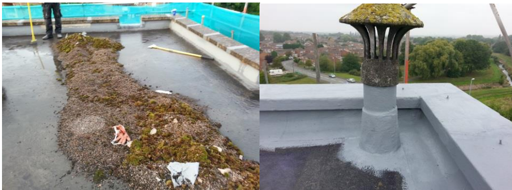
Removal of debris and vegetation
