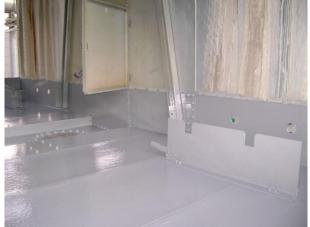
Completed application of chemical and corrosion resistant coating
