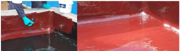
Fig 7 and 8 - Belzona 4361 applied to a concrete bund area
