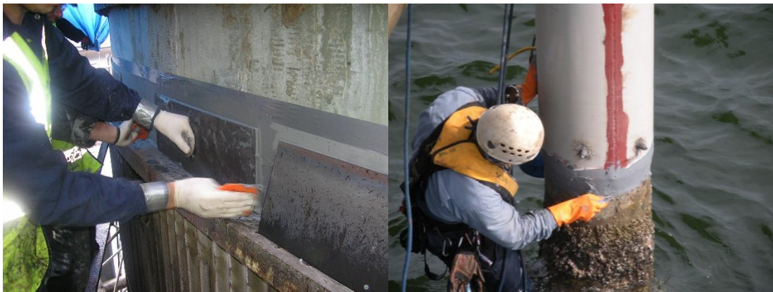
Belzona cold plate bonding in action
