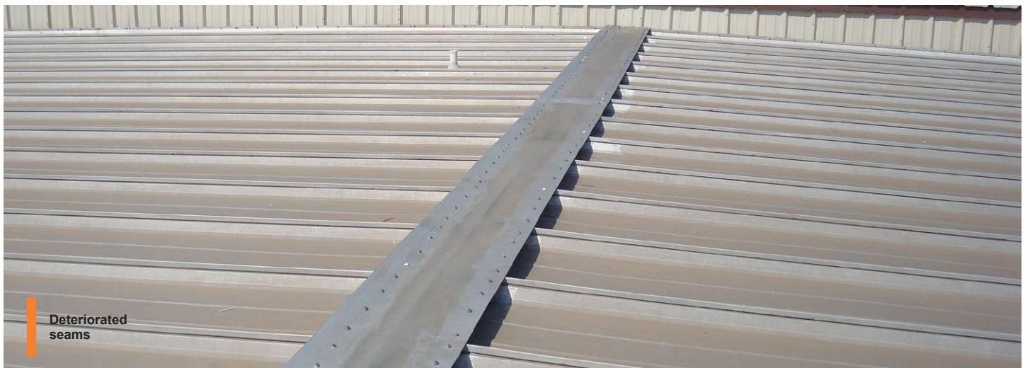
Leaking seams leading to water penetration
