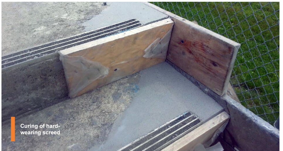
Wooden forms ensure correct shape achieved
