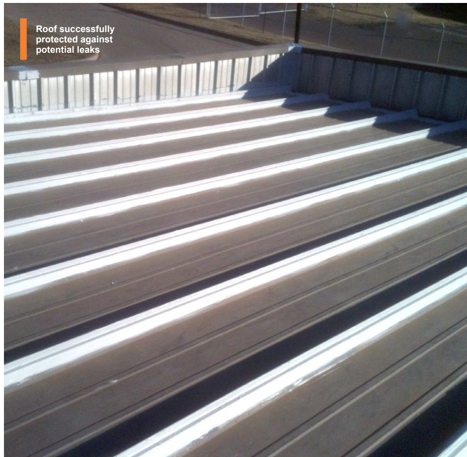
Seams sealed with breathable membrane
