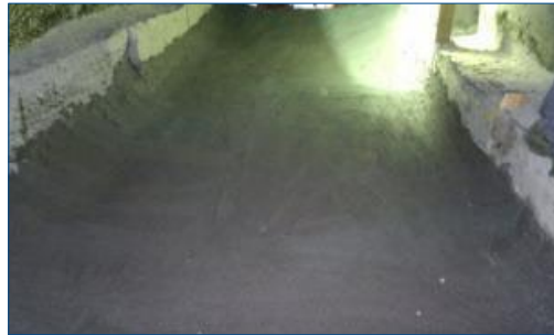
Completed application on a channel
