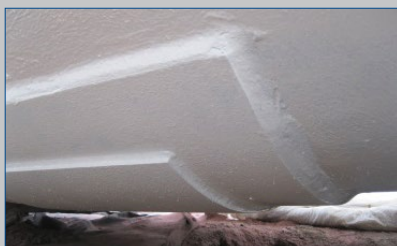
Pipe wear pads bonding
