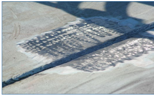
Surface ready for Belzona application
