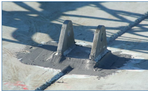
Bracket bonded with Belzona 1111
