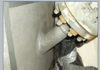
Corroded nozzle
