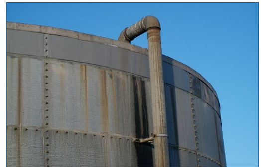
Tank repair completed
