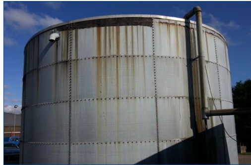
Corroded tank
