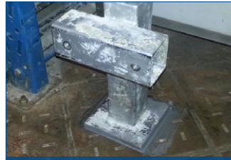
2. Load bearing shim creation
