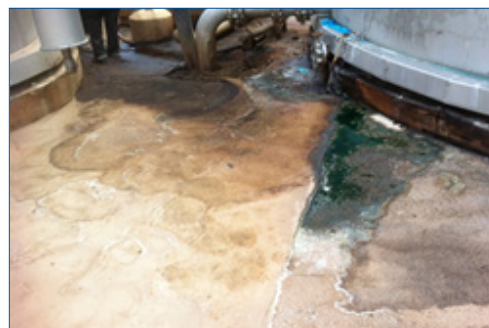
Acid attack at 49°C/120°F
