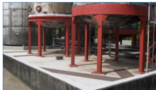
Concrete substrate repairs
