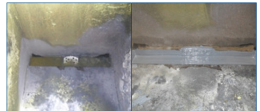
Through-wall damage repaired on pickle tank containing 36% hydrochloric acid
