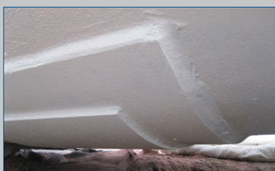
Pipe wear pads bonding
