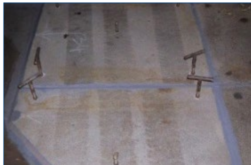
Plates bonded onto the deck
