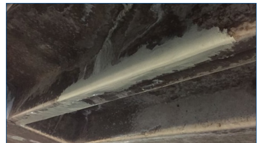
Rebuilding of overhead concrete
