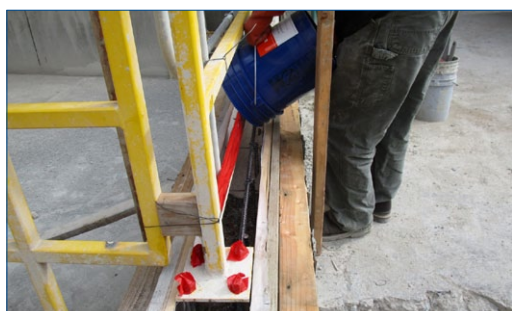
Removal of all deteriorated concrete
