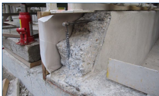
Removal of all deteriorated concrete
