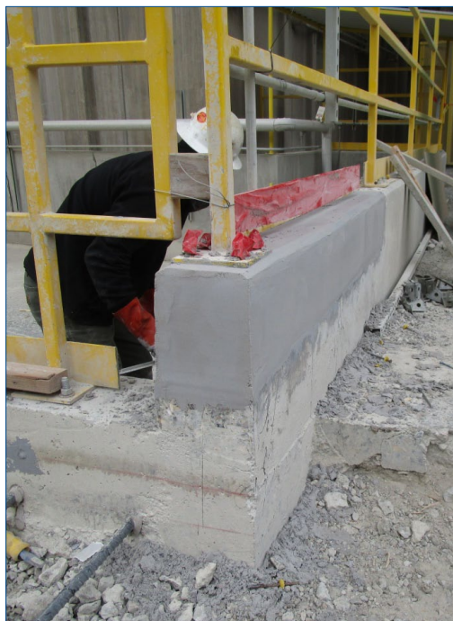
Secondary containment wall rebuilt and finished with a layer of Belzona 4111
