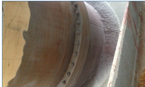
52" flange grit blasted
