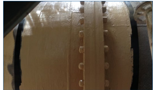
First layer of Belzona 3411 applied
