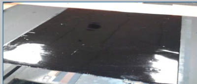
6. Finishing top coat applied
