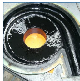
Localised repairs performed
