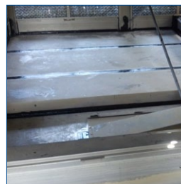
Sealing of cooling tower seams
