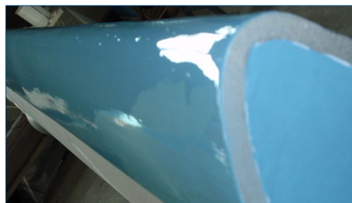
Belzona 1341 applied
