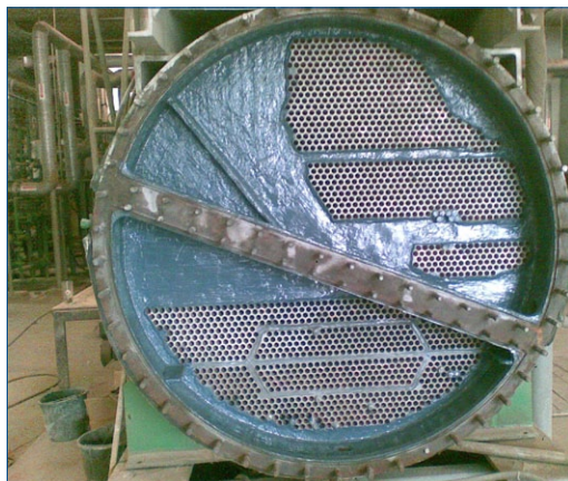
Completed coating of the tube sheet
