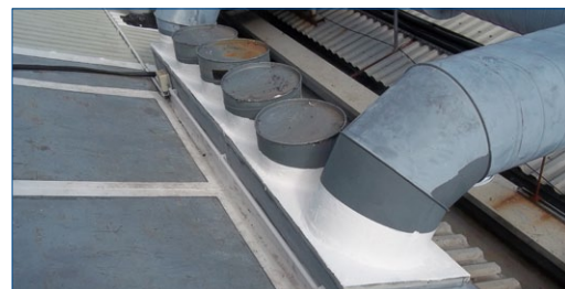
Completed sealing and protection
