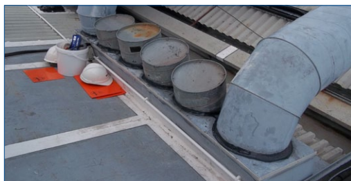
All joints sealed with Belzona 2211
