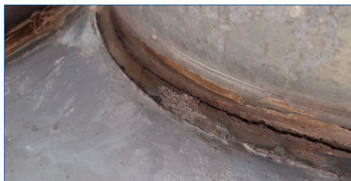
Deteriorated joint
