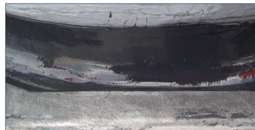
Belzona 2211 applied to seal gap
