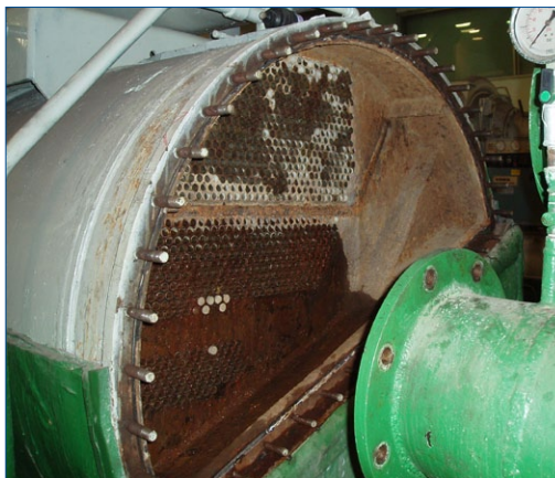
Tube sheet before application
