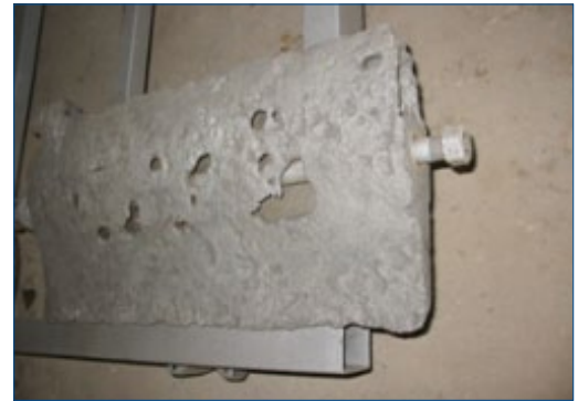
Blade after grit blasting
