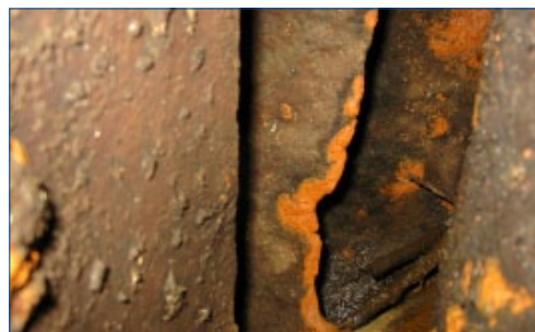
Fig 2: Deteriorated turbine runner
