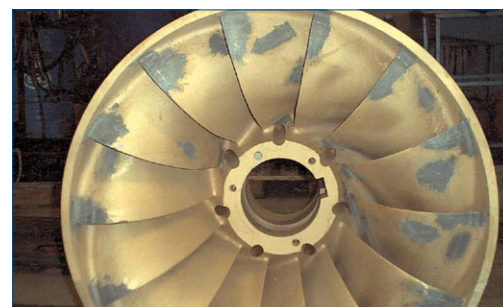
Application of Belzona 1341 (Supermetalglide) in progress to runner
