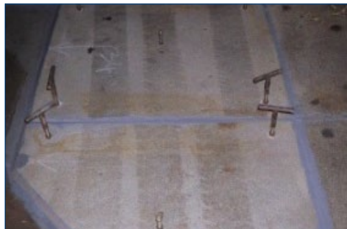
Plates bonded onto the deck
