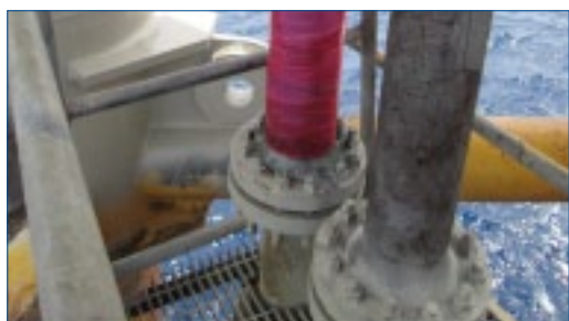
Belzona 9382 applied to consolidate repair
