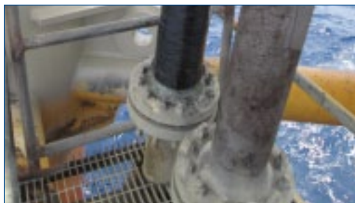
Four wraps of Belzona 1982 applied
