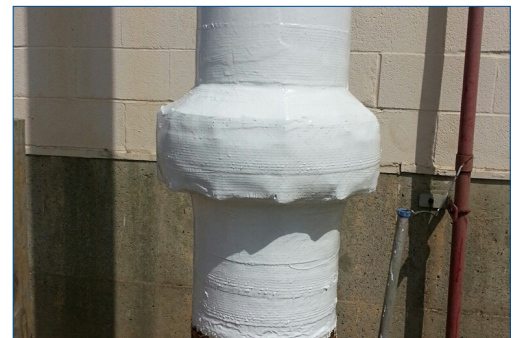
Encapsulated flange
