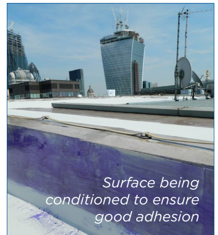
First coat of Belzona 311 applied
