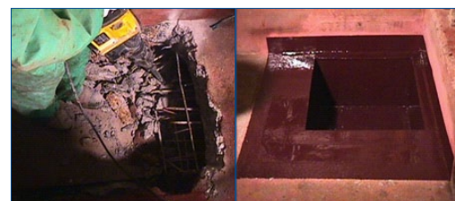
Badly deteriorated acid sump repaired
