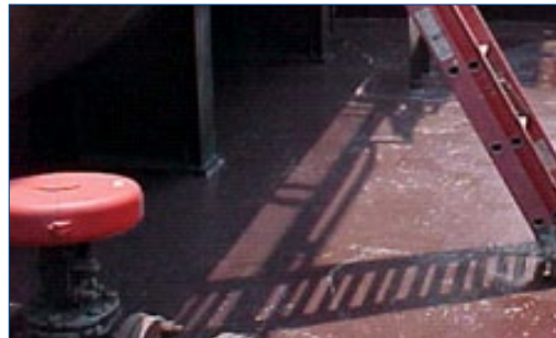
Coated area after eight years in service
