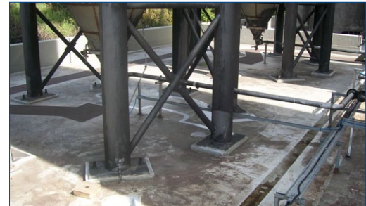
Concrete substrate repairs
