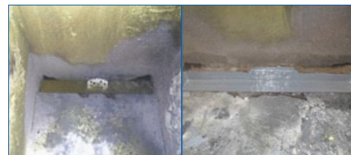
Through-wall damage repaired on pickle tank containing 36% hydrochloric acid
