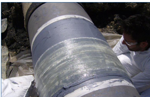
Reinforcing with resin soaked wrap
