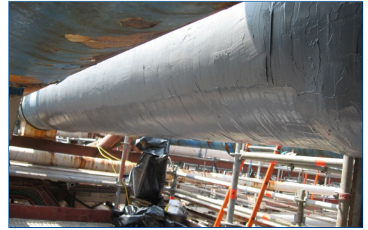
Belzona 4301 (CR1) for chemical resistance
