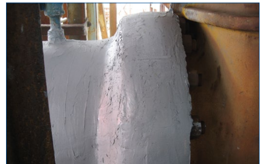
Belzona 1831 (Super UV-Metal) flange sealing
