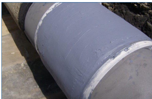
Applying polymer base
