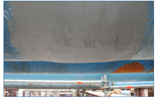
Temporary wrap to holed area
