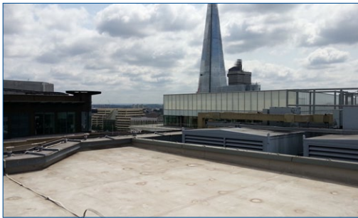
Roof cleaned and prepared
