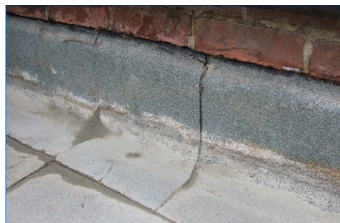
Leaking joints
