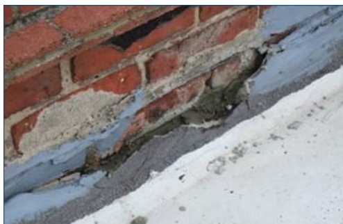
Deteriorated flashings
