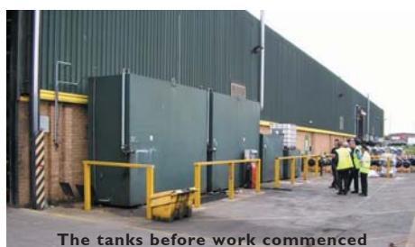
The tanks before work commenced
