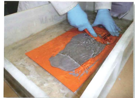
Description of Attached Image 2 – Under Water After application to the surface, a brush is used to work the Belzona 1831 mixture onto the surface to disperse surface oil and/or water before building up to the required thickness.
