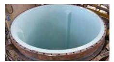
The light colours of Belzona 1593 allow easy visual inspection in vessels.
