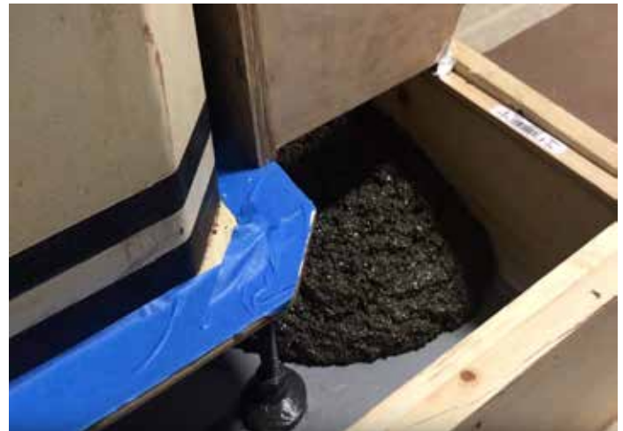
Belzona 7211 poured into place
