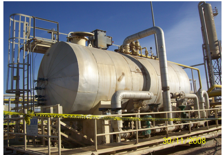
Belzona 5892 used to line a desalter
