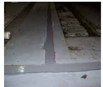
Repaired with Belzona 4521
