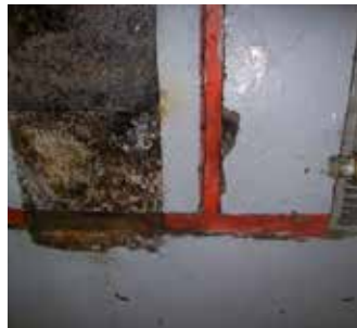
Deteriorated joint
