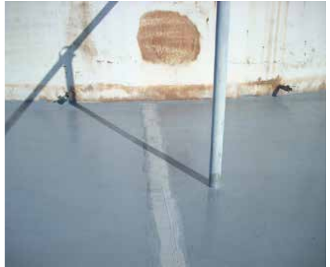
Used to refurbish failed joints in containment area
