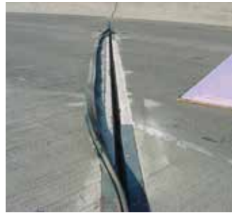
Damaged joint
