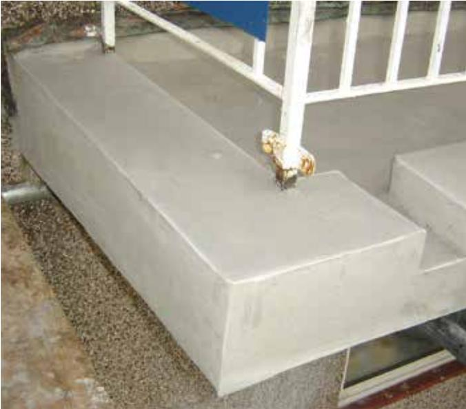
Belzona 4111 (Magma-Quartz) is a multi-purpose repair composite for the resurfacing, rebuilding and protection of concrete and stonework.
