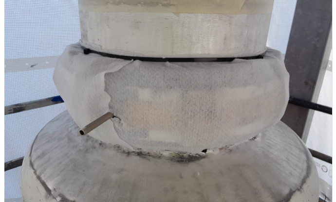
Prepared flange, ready for application
