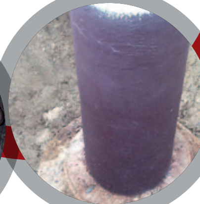
Repair of Thin Wall Defects
