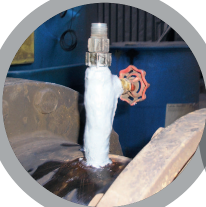
Leak Sealing of Pipework
